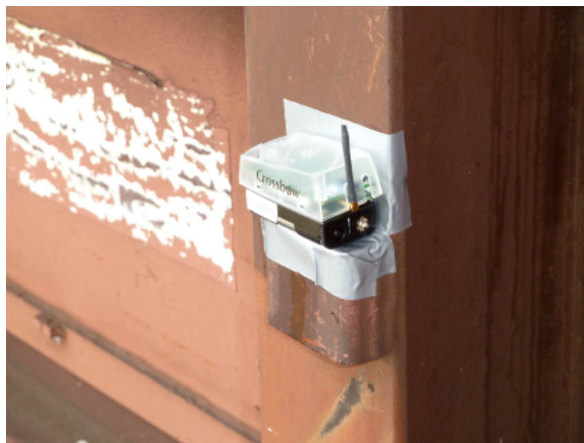
Figure 34 Box for sensor's protection
