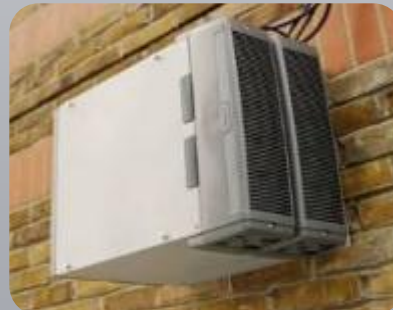
Outdoor building walls & rooftops
